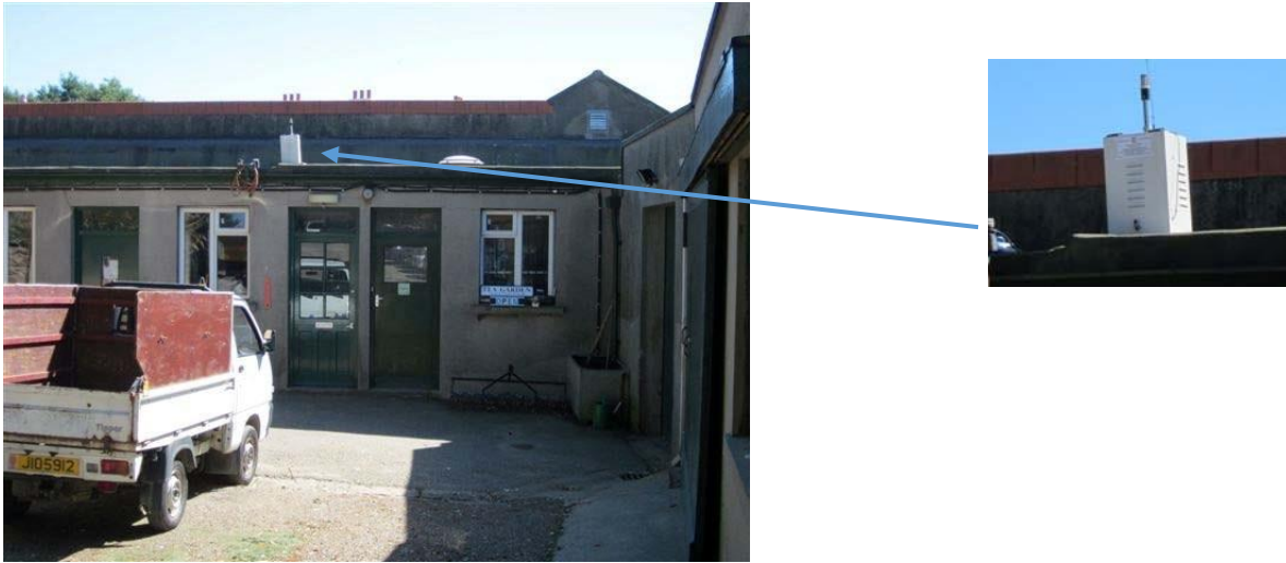
Photograph 3: Position of the Osiris unit at Howard Davis Park
