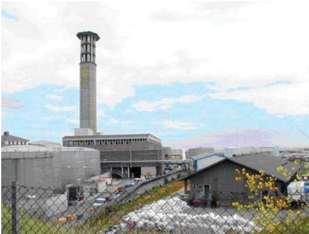
Photograph 2: The Jersey Electricity Company power station.
